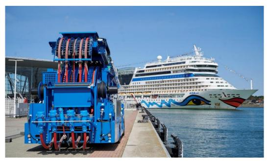
Fig. 6.8. The shore power facility in the Warnemünde cruise terminal
